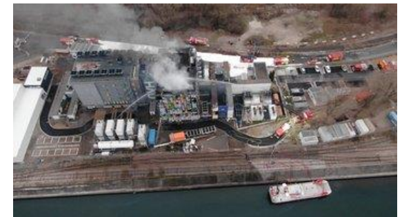
DRC-EB-001 trial - OVD data centre fire, Strasbourg 2021
