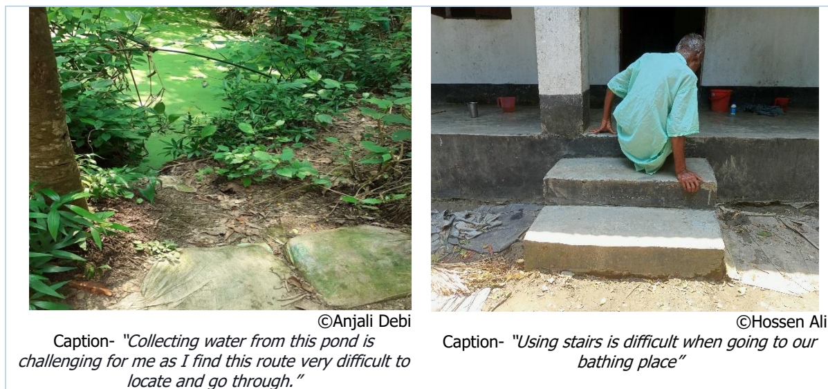
Figure 35: PhotoVoice images of the non-inclusive entry path of the bathing place for persons with disabilities and older people
