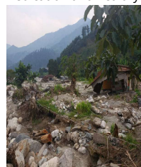
Figure 2: Section of Kilembe Hospital destroyed by floods
