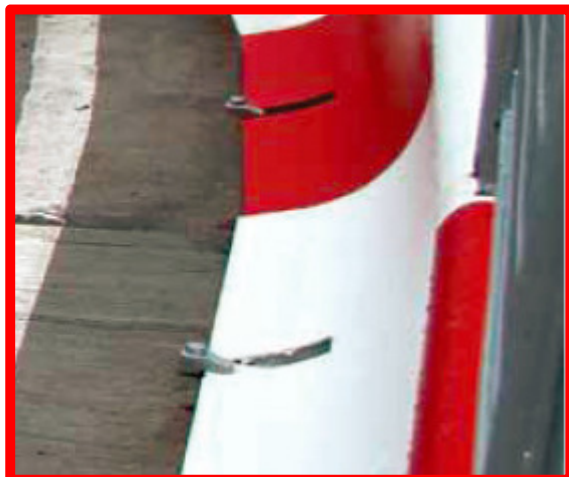
Figure 3 - Mass barrier mechanically fixed to carriageway.
